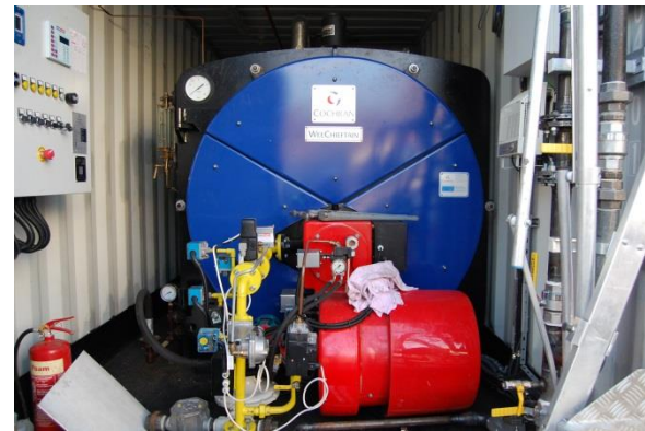
Steam Boiler Conversion
