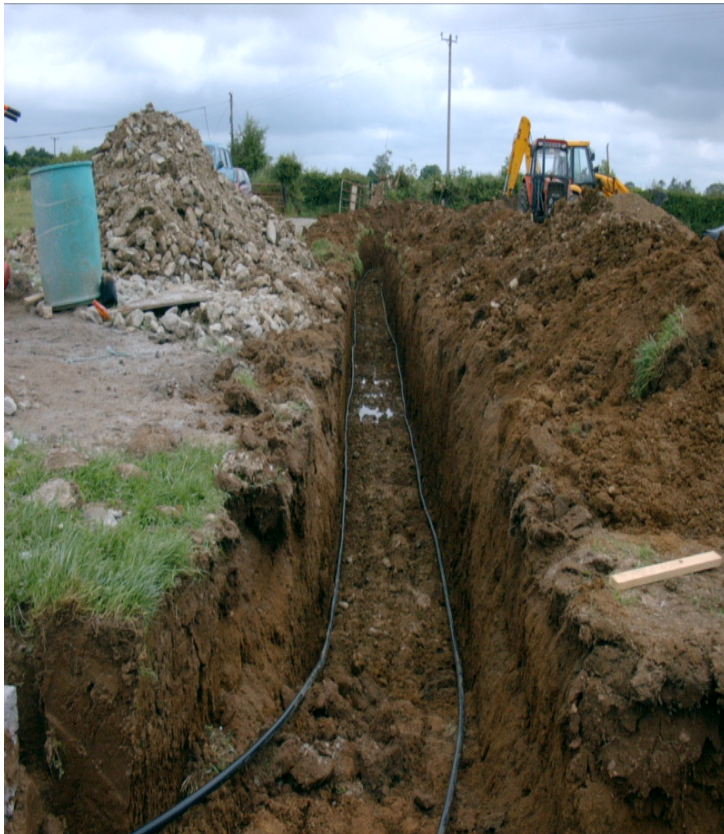
Installation horizontal collector:
