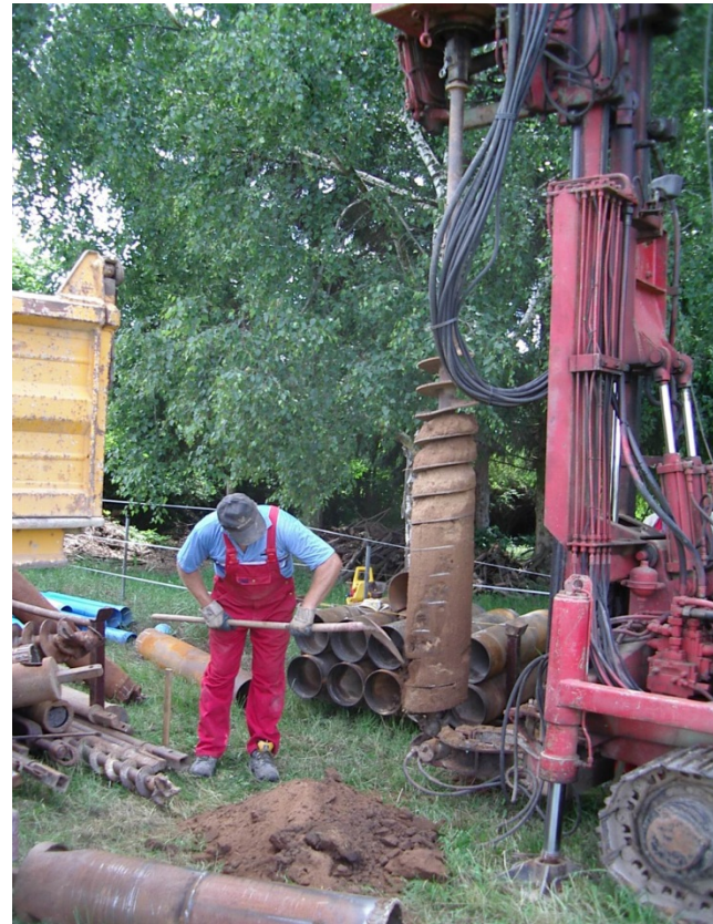
Installation vertical collector:
