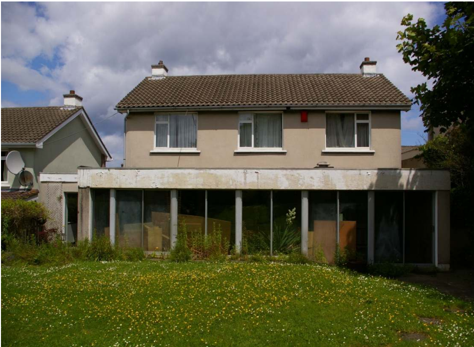
REAR VIEW OF HOUSE : PRE-REFURBISHMENT
